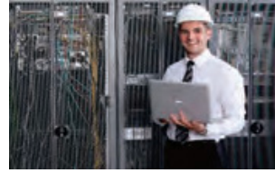
Traditional Server Room
